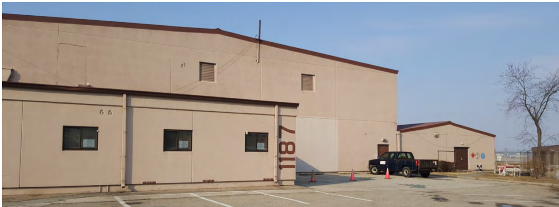
Fig. 12: Bldg 1187, parking and entrance area (door by the truck)
