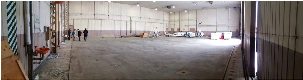
Fig. 17: Bldg 1161, King Air aircraft hangar floor, lab space.
