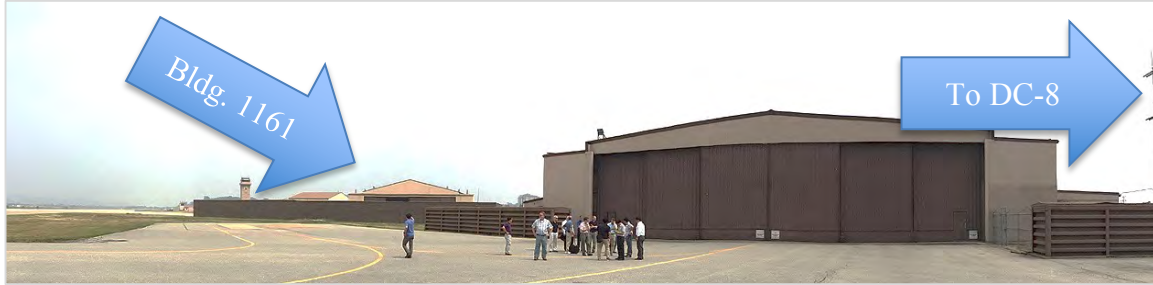
Fig 14.: Ramp view of Bldg. 1187.
